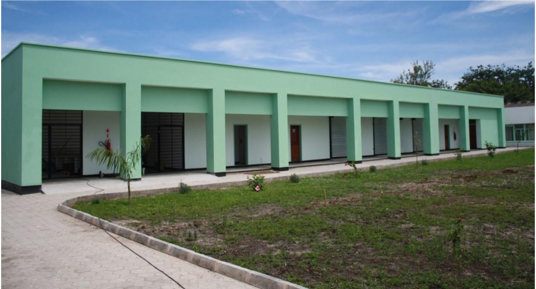
Maintenance Building – Side/Front View
